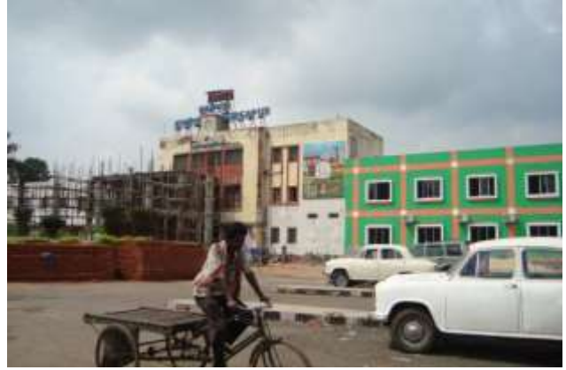
Durgapur Station Entry
