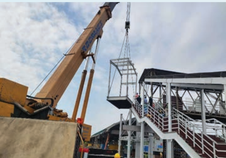
Placement of top head on the pre-fabricated staircase
