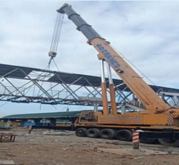
Removal of dismantled last span
