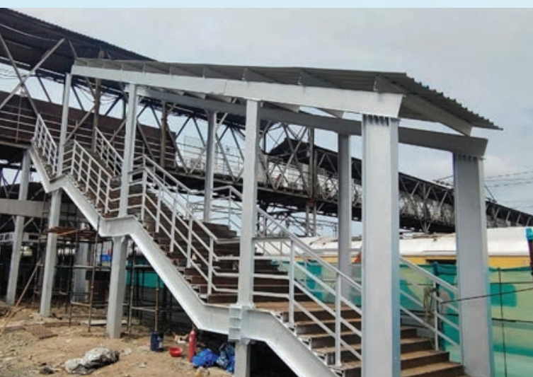
Pre-block staircase fabrication and construction
