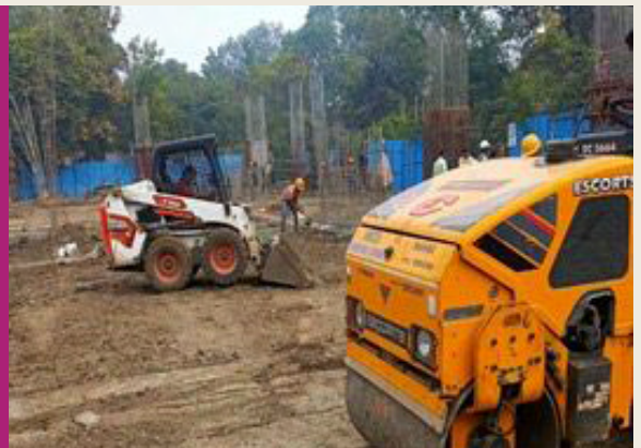
COMPACTION ROLLER 5MT FOR COMPACTION OF SOIL AND BOBCAT FOR BACKFILLING OF SOIL
